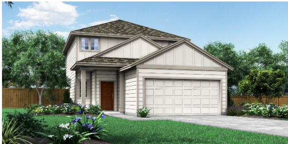
Stonewall C with siding
